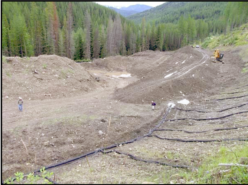
Figure 15. Shell Canada Ltd.'s Wheel Creek CBM site, collapsed and slumped into Wheeler Creek in heavy rains, southeast British Columbia, Canada. Photo by Erin Soxton. (From Flathead Basin Commission).
