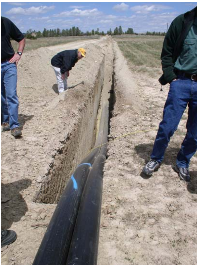
Figure 6. New pipeline being laid in the Powder River Basin. One line carries methane, and the other transports product water away from the well.
