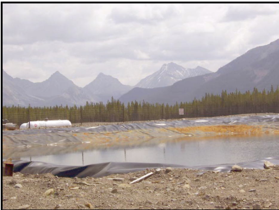
Figure 14. Encana/StormCat wastewater settling ponds at exploratory CBM well site. (From Flathead Basin Commission).
